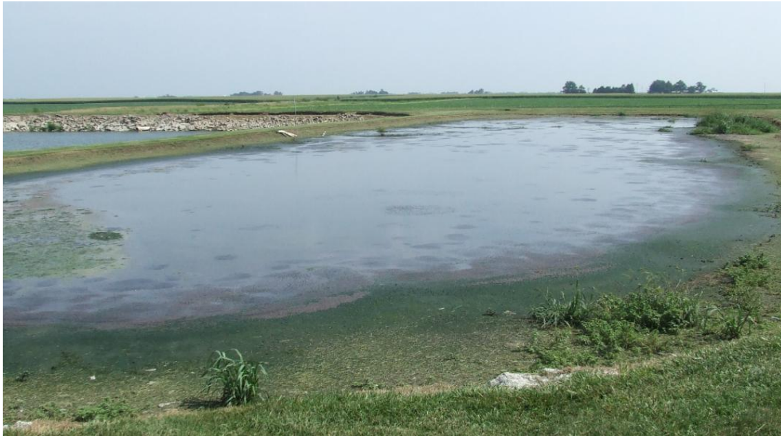
Figure 2-14 Sludge Storage Lagoon
