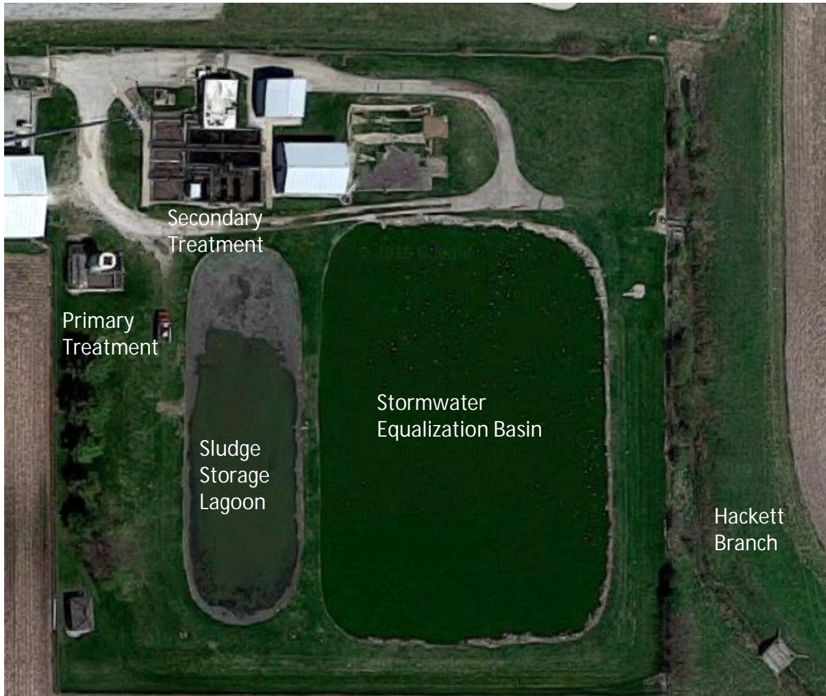
Figure 2-1 Tolono WWTP and Lagoon Aerial
