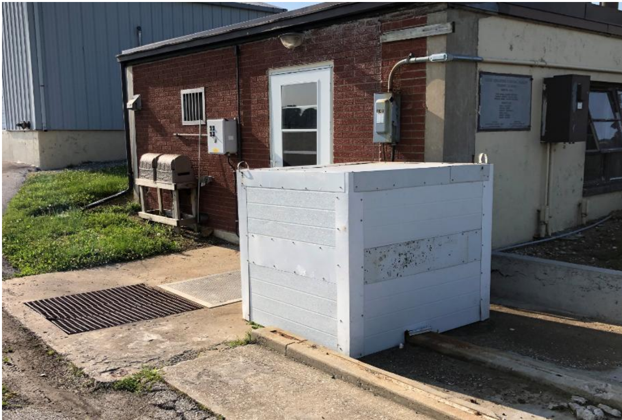
Figure 2-5 Influent Wet Well and Stormwater Pump and Cover
