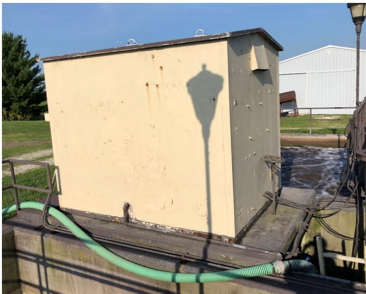
Figure 2-12 Chlorine Contact Tank with Chlorine Building
