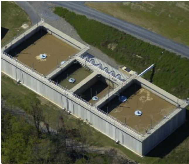
Figure 4-3 SBR Example Reactors Aqua-Aerobics
